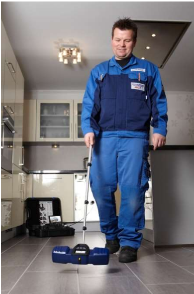
Fig. 7: Localizing the camera head underground
